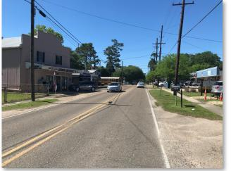
Figure 74. Existing Conditions along LA 21: No vehicle and pedestrian separation and designation, high speed traffic and no bike lane
