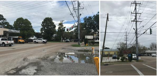
Figure 23. Existing Conditions. Poor drainage, undesignated egress and ingress, missing curbs and
